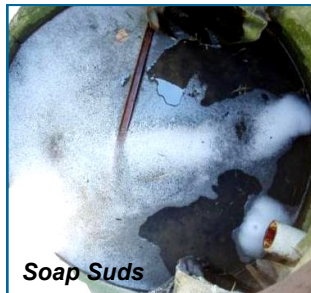
Broken Sanitary Sewer
