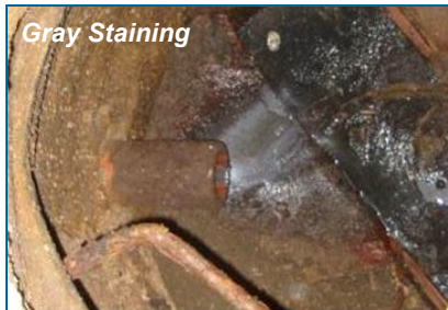
Broken Sanitary Sewer
